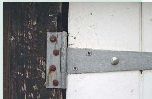
Rose-nailed strap hinge with coach-bolt through door
