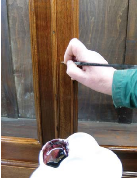
Doing the localised colouring out on the door stiles
